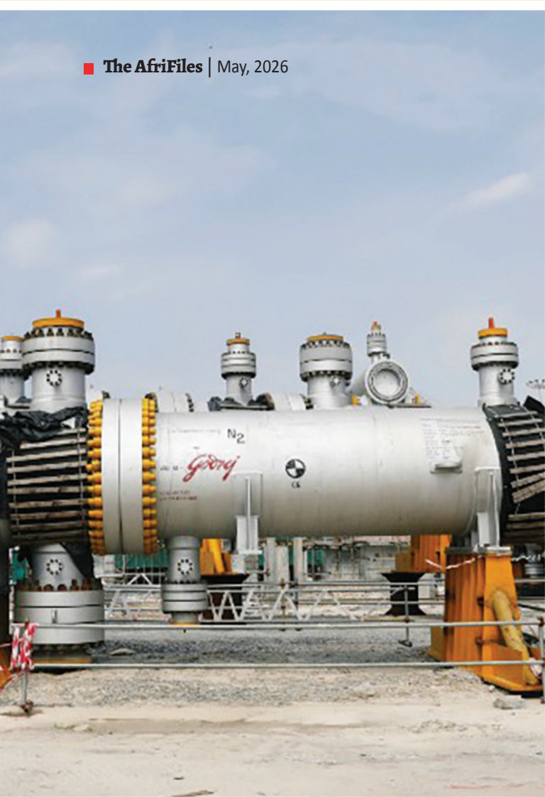
A view shows part of Dangote oil refinery in Ibeju, Lekki District, on the outskirts of Lagos, Nigeria. Photo: Temilade Adelaja / Reuters.
